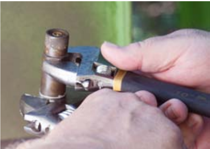
Tightening up renovated connector.
