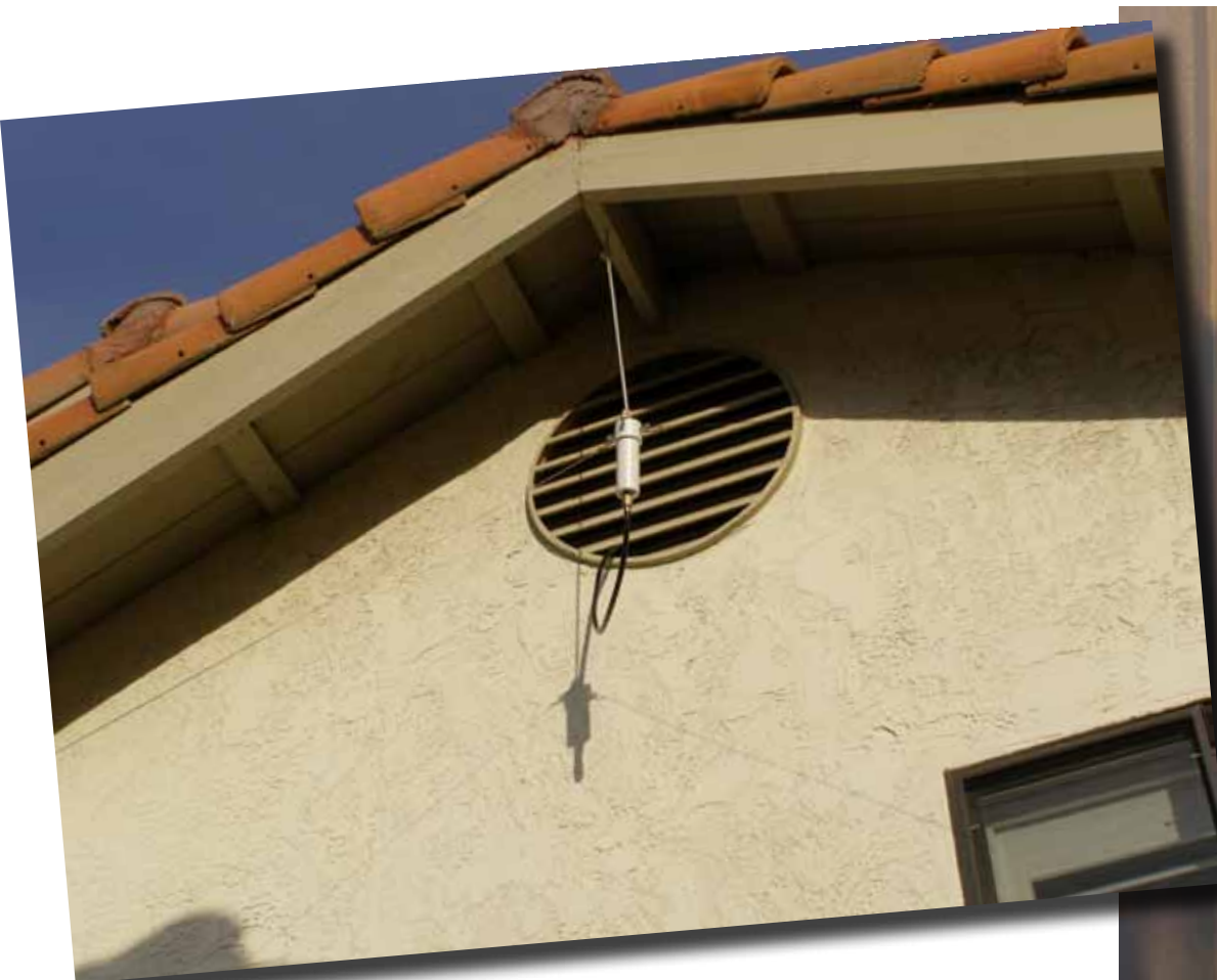
17 METER DIPOLE INVERTED VEE
