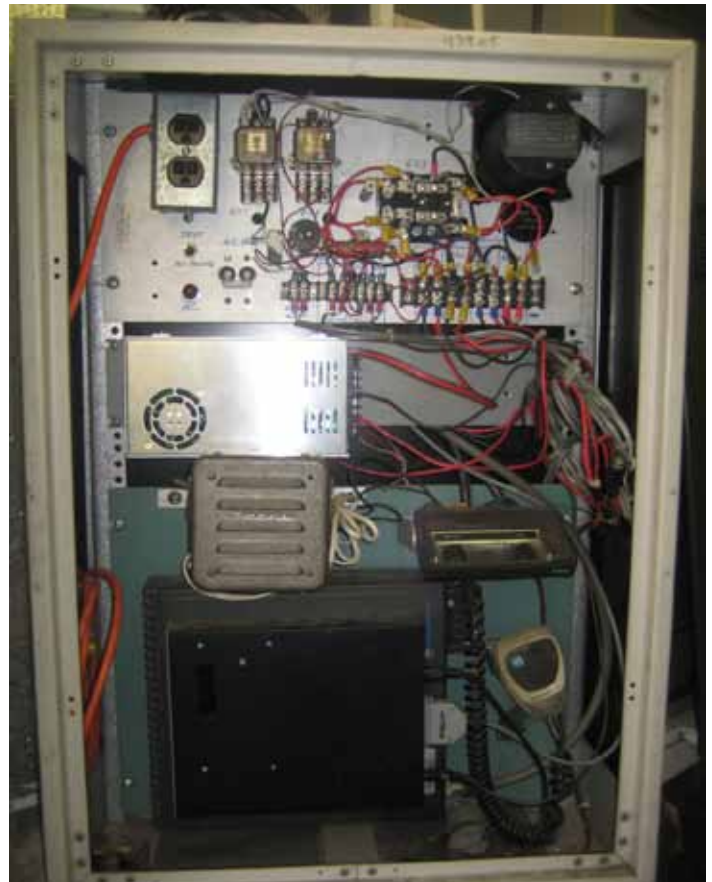
METRO NET WITH CONVERTER IN MIDDLE REPLACING LARGE POWER SUPPLY
