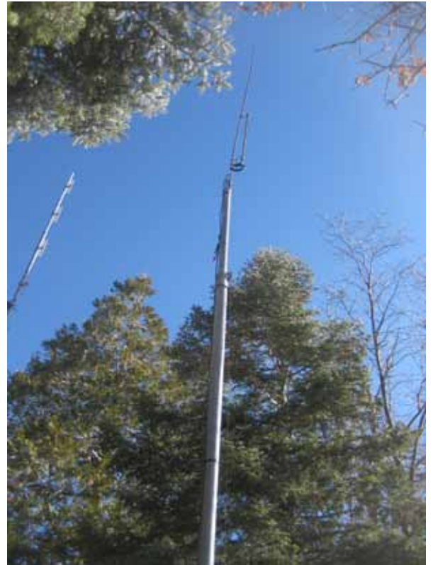
NEW 6M BENT ANTENNA ON FOLD OVER MA40 MAST
