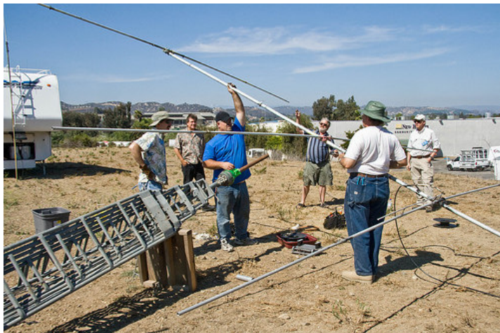
Preparing to mount a yagi antenna on top of a tower.
