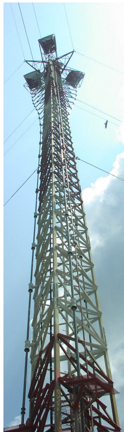
300 ft. microwave tower, owned by amateur radio operator AD5T in Mississippi.
