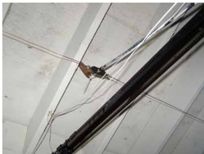
STEALTHY CENTER-FED DIPOLE AT KJ6SJZ
