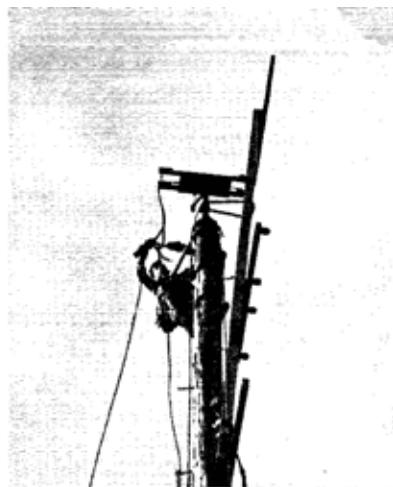
The boom is raised by block and tackle after the cradle is in place on top of the pole. In this view, the boom is on the way up and a rope is being tied to the boom so that it can be pulled into place over the cradle.
