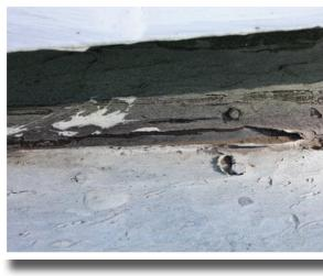
This leak allowed water to seep into the sub-roof of the building and eventually drip down directly upon the 6 meter repeater. This failed seal was stripped and redone in order to provide weather proofing for the rains that fell starting Sunday night (photo in center). The emergency water ducting previously erected in De-
