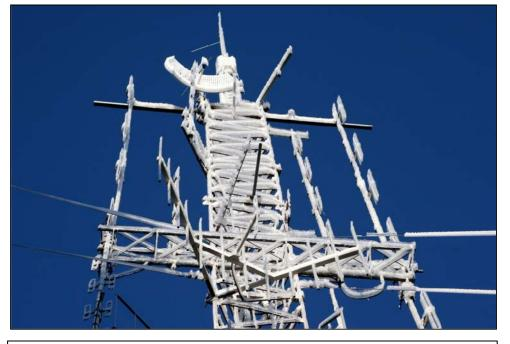
W6NWG in mid-January 2007h some snow and ice loading on the tower. Photo W5NYV. Designing a tower installation requires consideration of both wind and snow & ice loading. Although some minor damage was sustained in the March of 2006 snowstorm, no damage was noted during the January precipitation.
