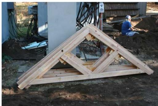
Above, framed pieces ready to go up on top of the freezer building. Wood was cut, framing accomplished, and the pieces all put together at the repeater site. KC6YSO in background.
