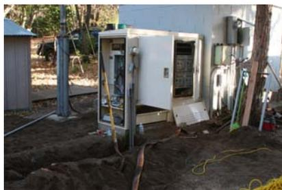
Above, the power upgrade work is in process. In this shot one can see the several cabinets that contain the equipment used to distribute power to the buildings at the site as well as trenches for conduit. At right, roof is constructed by Jim KF6RFW. Photos by W5NYV.
