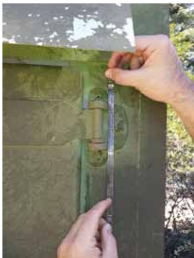
Hinge needs replacing. Photo by WA2OOB
